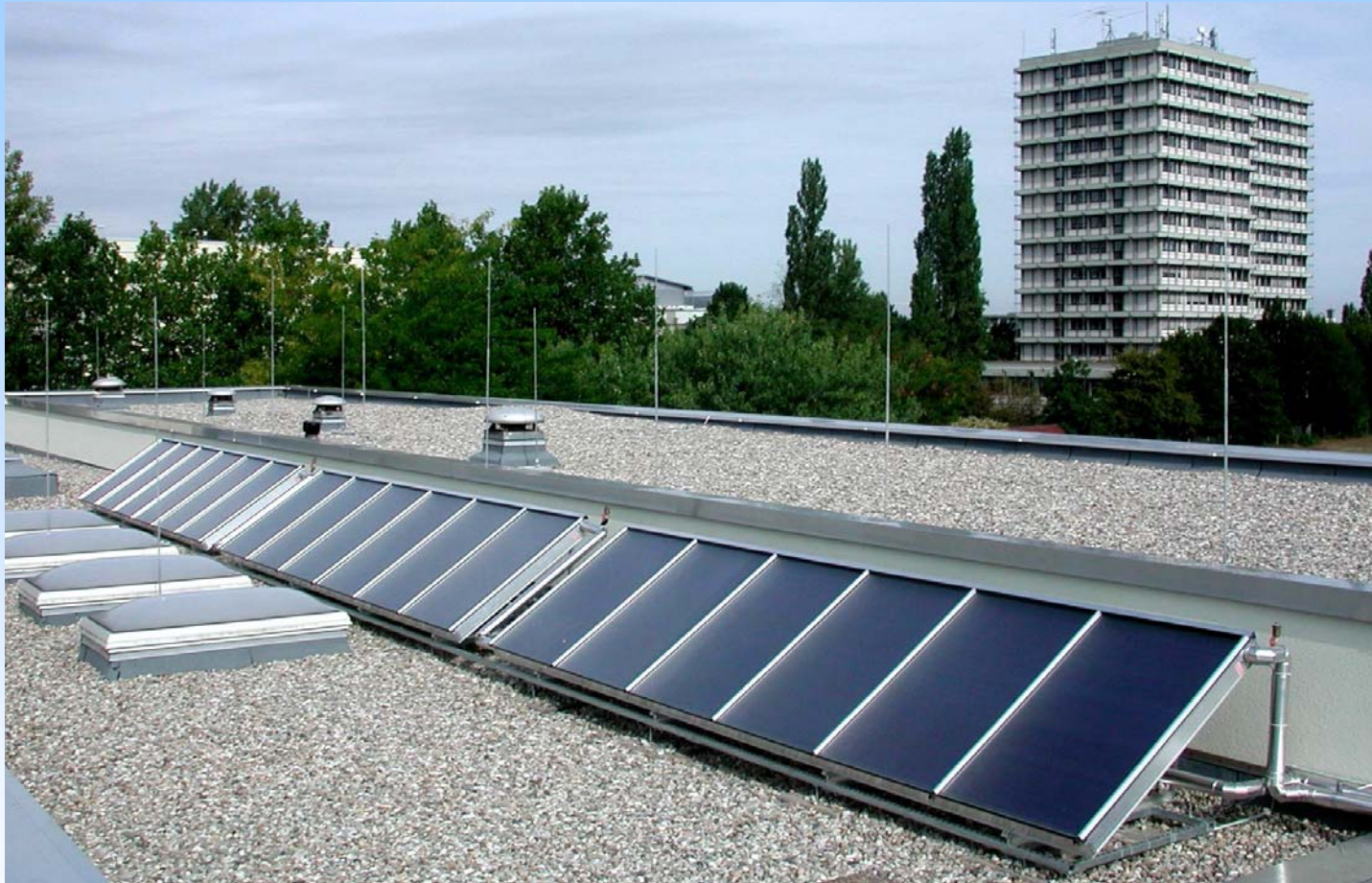
Solar thermal system at Marie-Baum school Hot water for the kitchen
