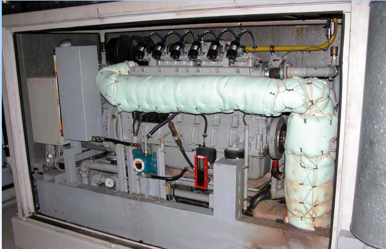
Small scale cogeneration of heat and electrical power with an gas motor generator unit in an sports center in Heidelberg
