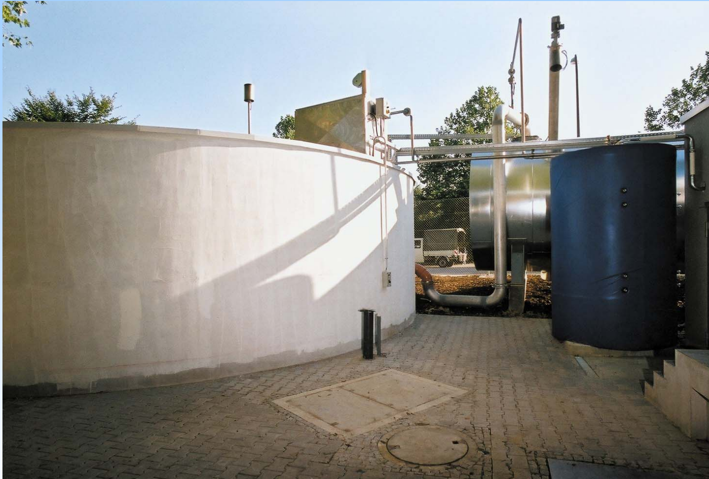
Biogas system with CHP unit at the Heidelberg Zoo
