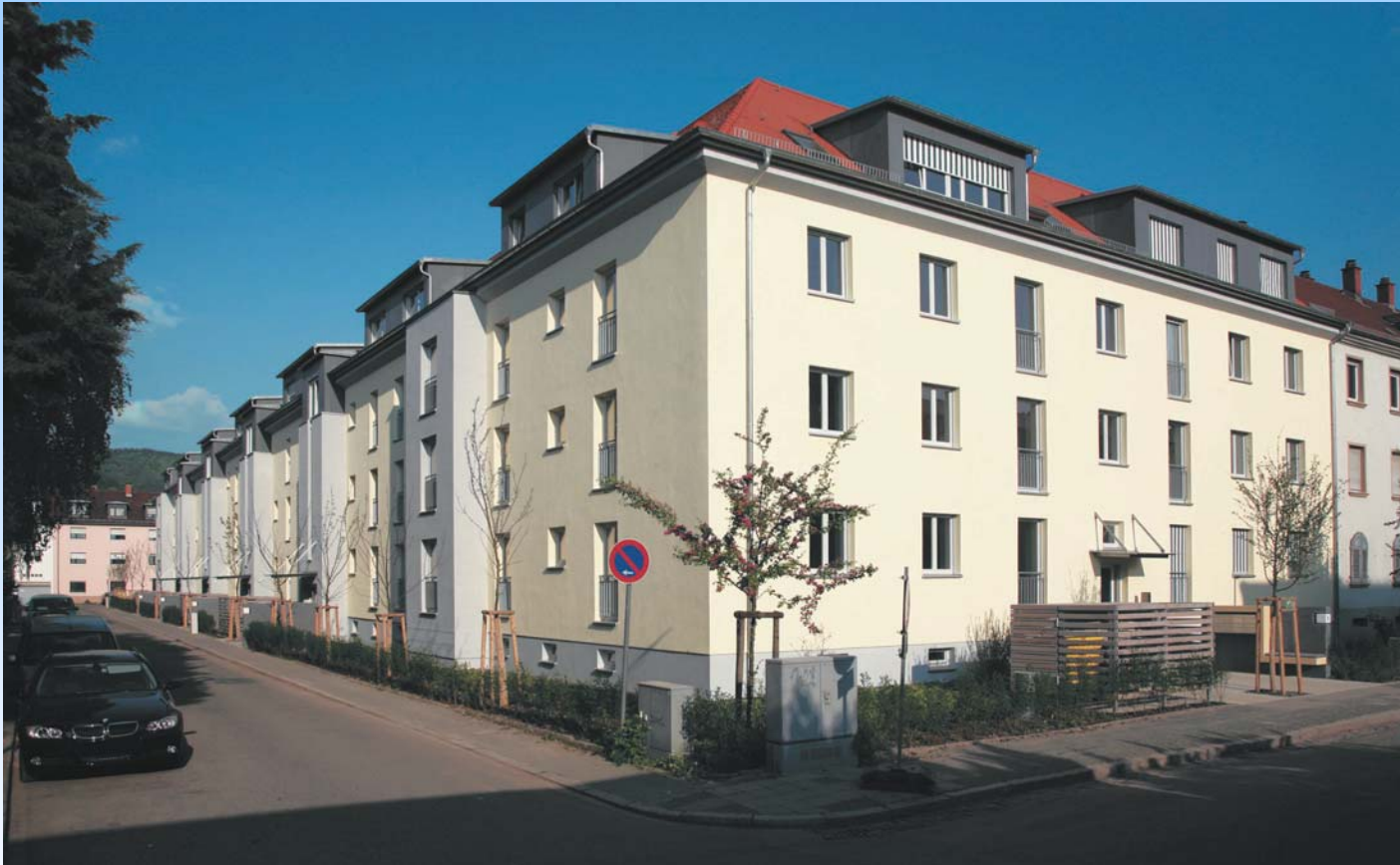
Retrofittet residential houses „Blaue Heimat“ of the Heidelberg municipal housing society GGH Heat demand reduced from 187 to 21 kWh / m 2 a
